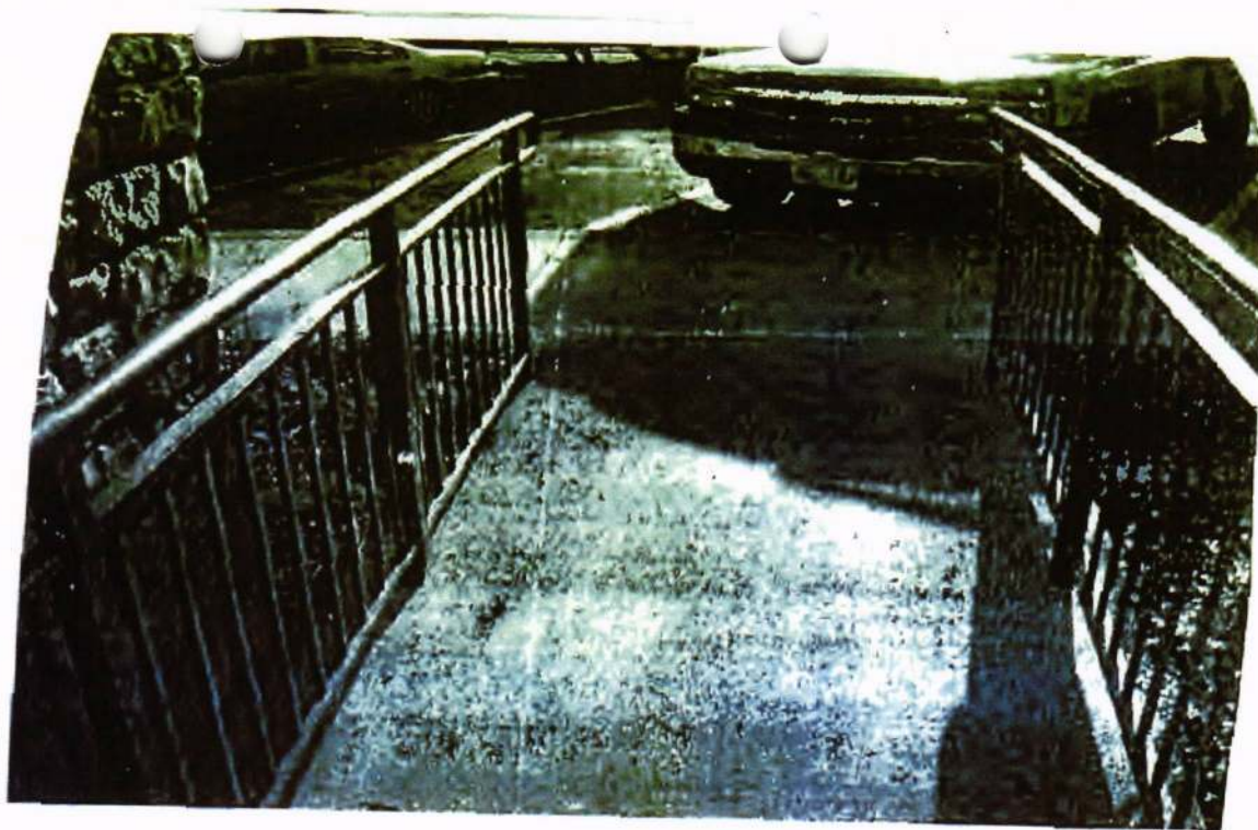
Figure 1: Sidewalk/Ramp Approaching the Parking Lot Area
